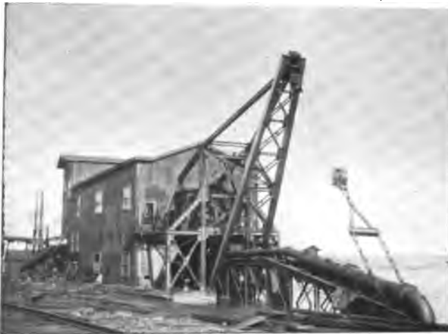
B. THE LARGE DREDGE FOR HOISTING THE CALUMET AND HECLA STAMP SAND FROM TORCH LAKE.
